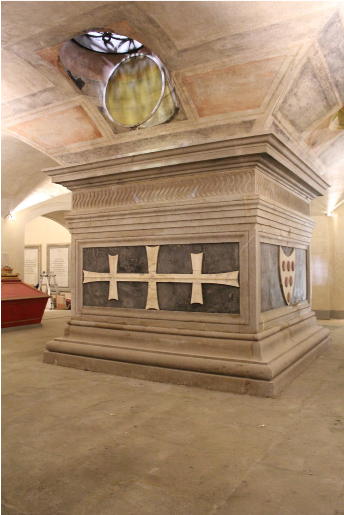
Fig. 8: Burial chamber of Cosimo il Vecchio, connected to the floor slab above in the nave of the church, seen in figure 15. Image: S. Cantell, Florence, 2022.
